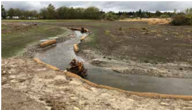
Restored meandering creek. Soon native plants will line the banks.
