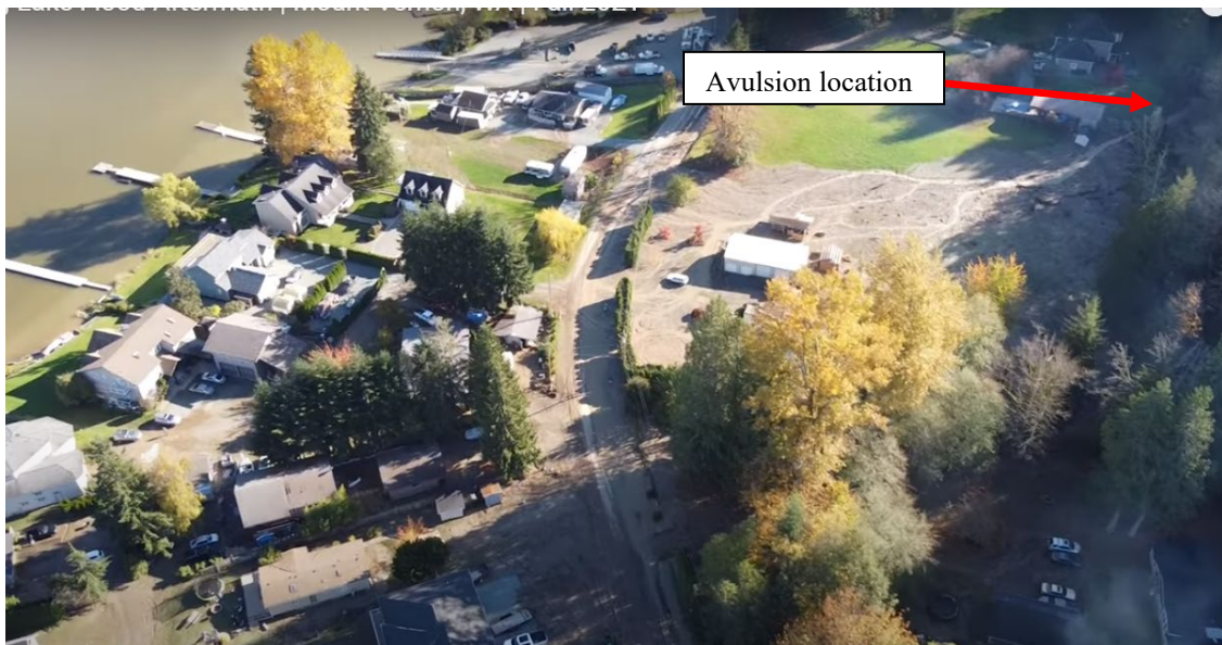
Figure 19. View of flooded area showing the avulsion location and area where flood water spread across the alluvial fan.
