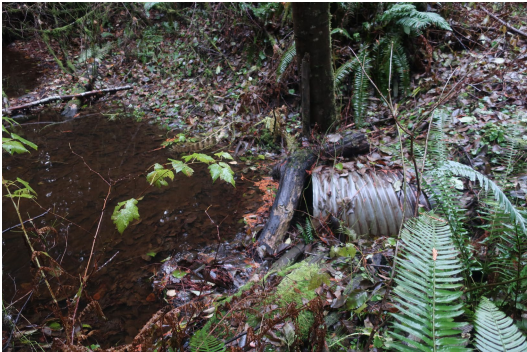
Figure 10. Culvert inlet at old logging road
