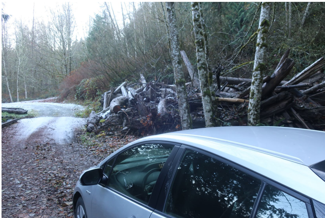
Figure 2. Large wood debris jammed at bridge West Lakeview Lane at the apex of the alluvial fan.
