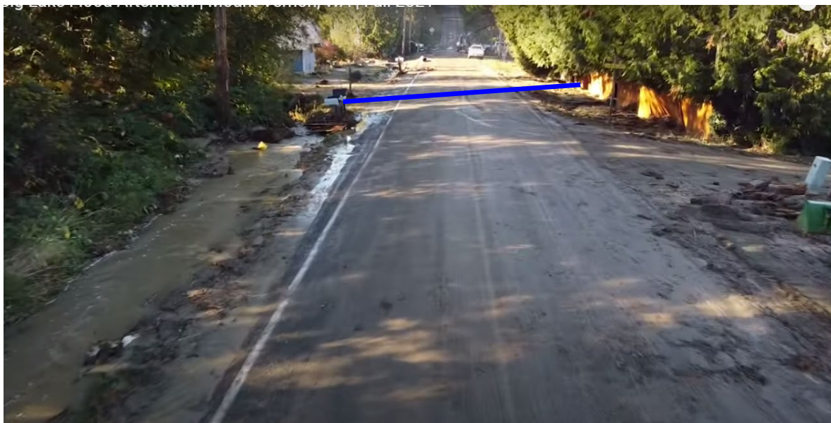
Figure 21. View of water flowing in ditch to stream culvert indicated as blue line across road.
