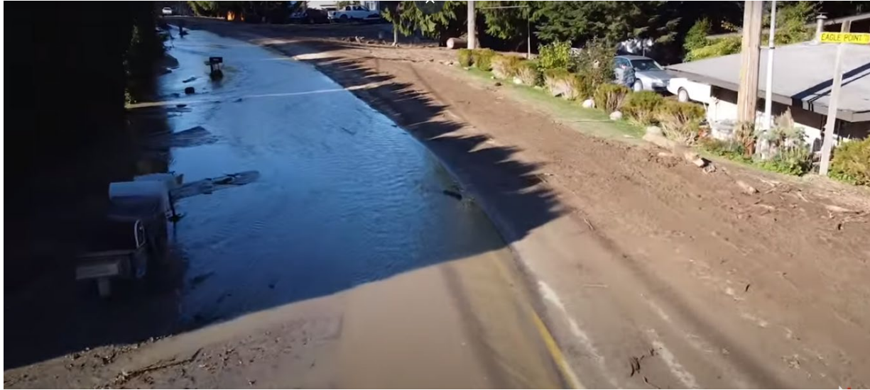
Figure 20. View of water flowing in ditch and on road. Note mud from higher water showing areas where water flowed across the road to the properties on the east.
