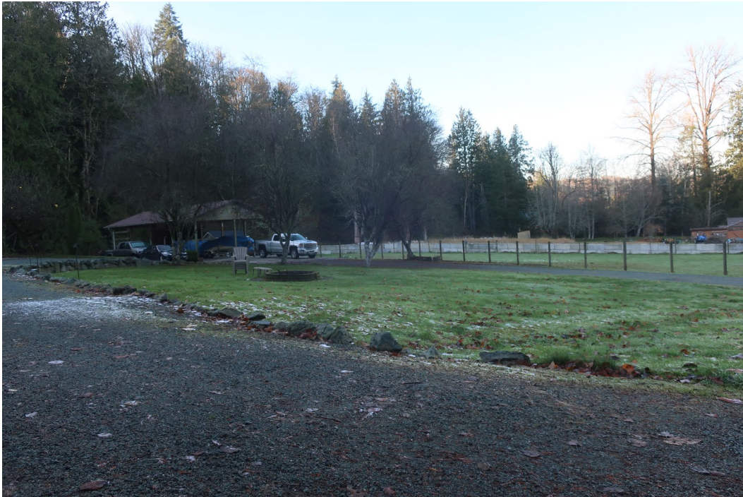
Figure 4. Overflow swale east of main stream which is located behind buildings.
