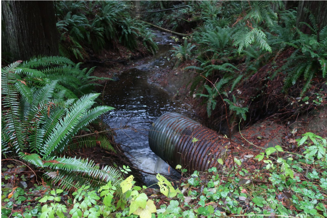
Figure 11. Culvert outlet at old logging road
