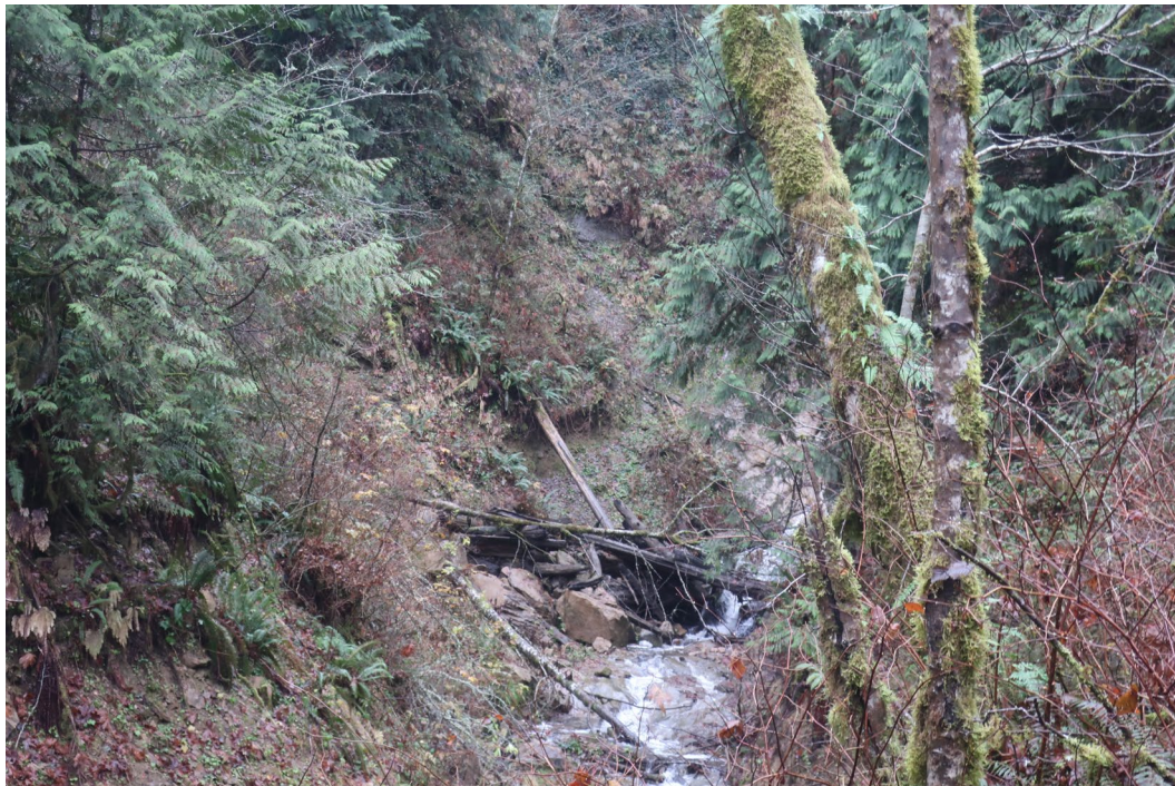
Figure 14. Shallow bedrock slide in steep narrow bedrock canyon
