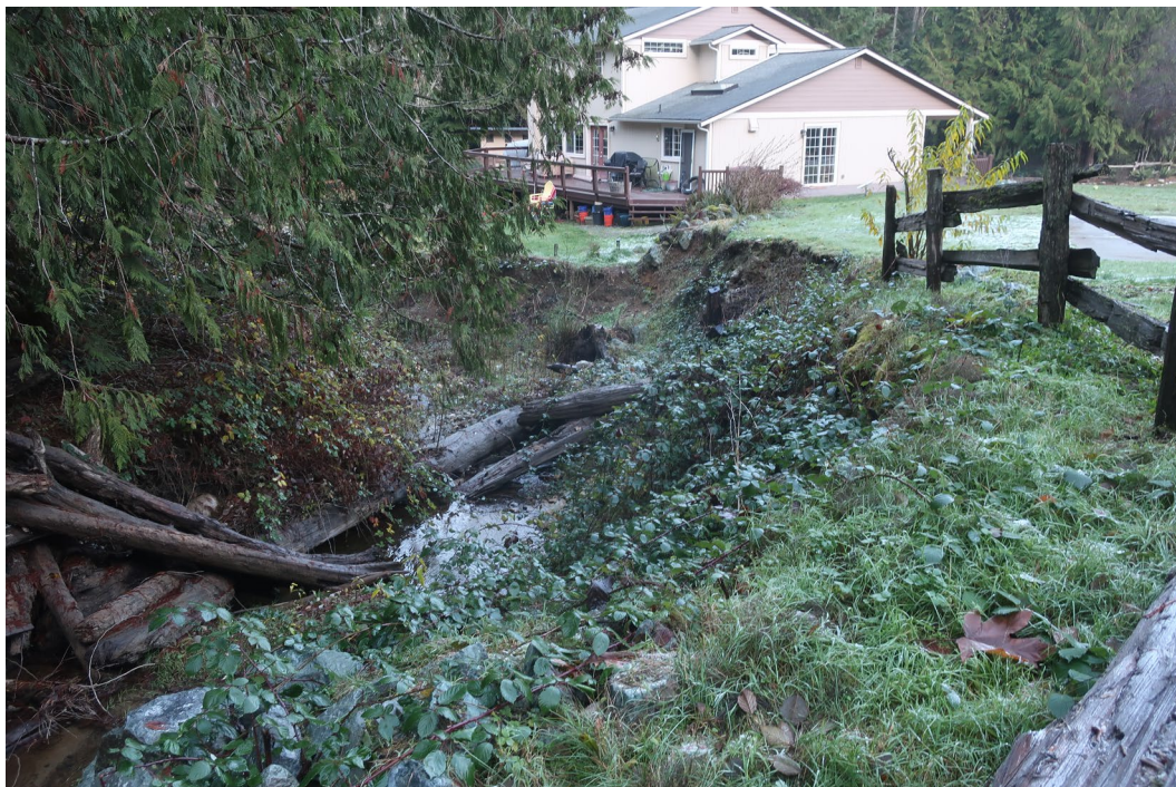
Figure 3. Deep incised stream reach on upper fan just below West Lakeview Lane bridge.
