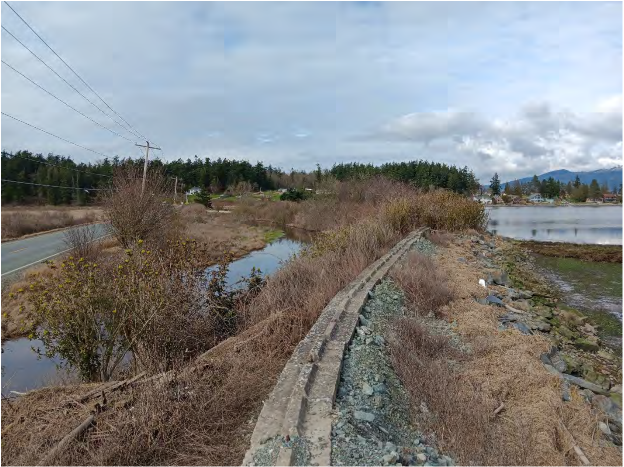
Figure A-15. View to the north along the eastern shoreline. Dike/armoring is in the center of the photograph and drainage channel is visible between the armoring and road to the left (March 2024 photo).
