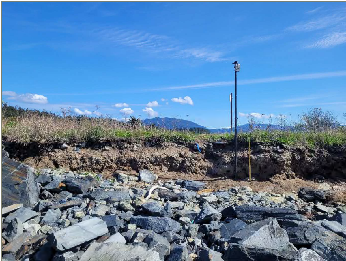
Exhibit 3-8: Dike Erosion at GPS Point L
