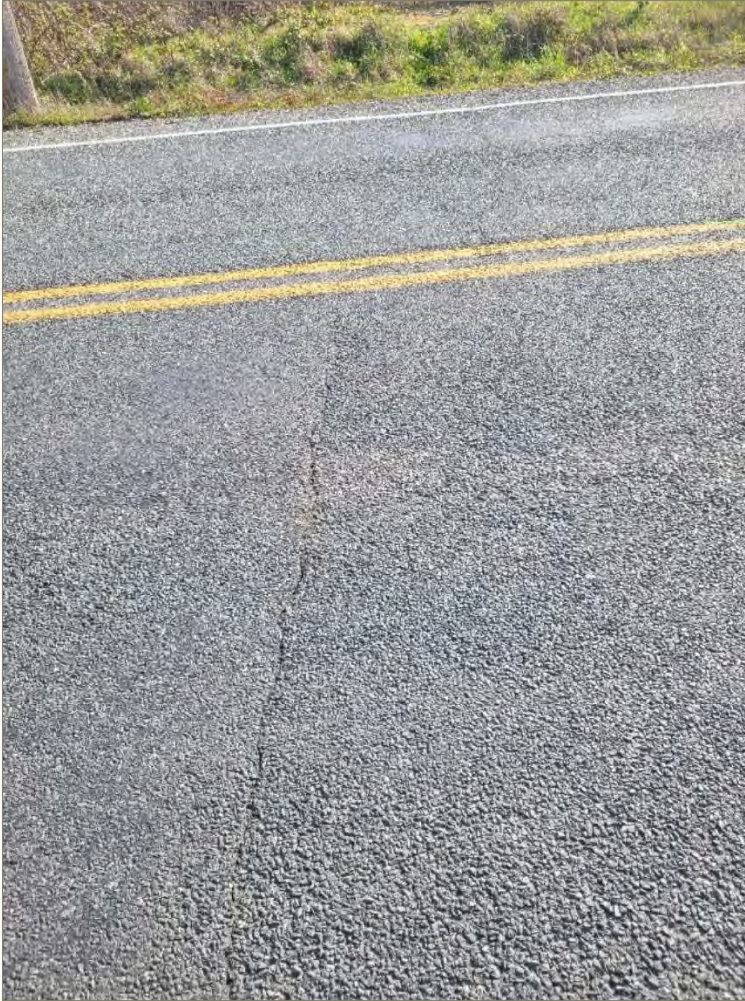
Exhibit 3-3: Transverse Crack in Samish Island Road
