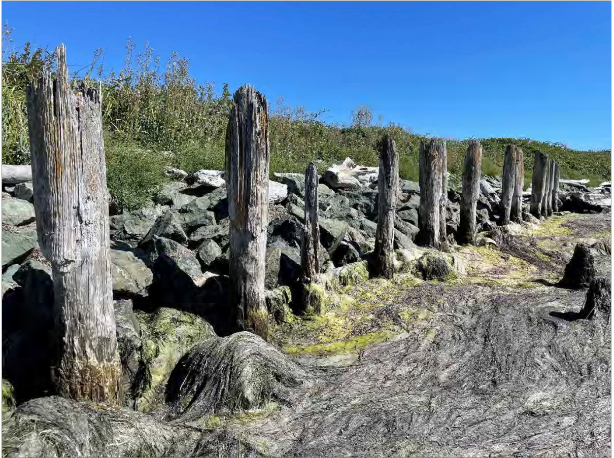
Exhibit 3-7: Piling Supporting Riprap
