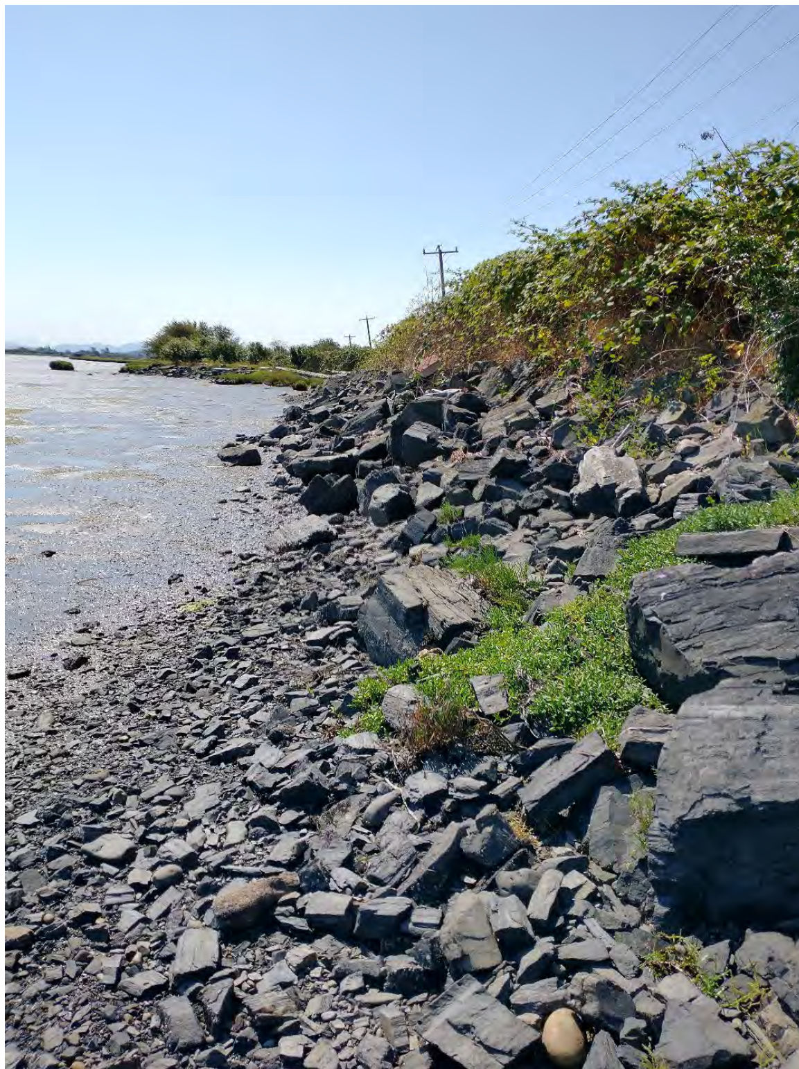
Figure A-5. Rock armoring along the eastern shoreline (July 2022 photo). View looking south.
