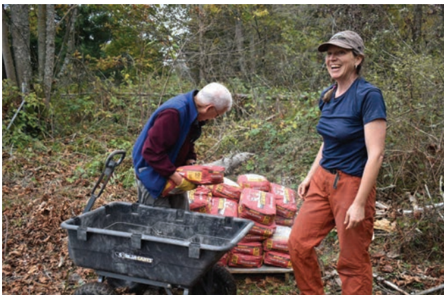
Sarah volunteering on the solar system installation at the March Point Heronry
